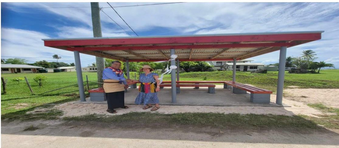
Bus Station at Ha'ato'u (Ha'apai) project, 2023
